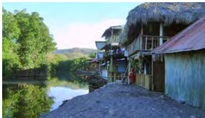
Typical tourist hotel, La Libertad, El Salvador. Wastewater is treated in septic tanks and discharged to surface water, resulting in environmental pollution.
