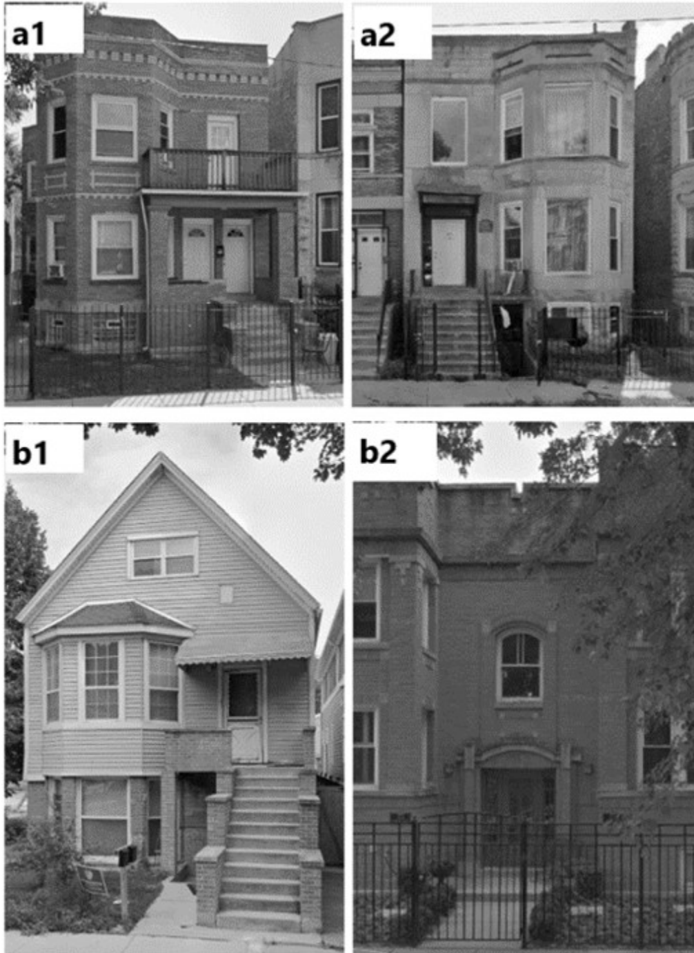
Figure 2. Google Street View images of sampled drop point units and substituted non-drop point units
