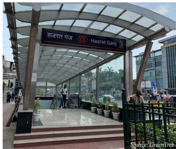
b) Lucknow metro
