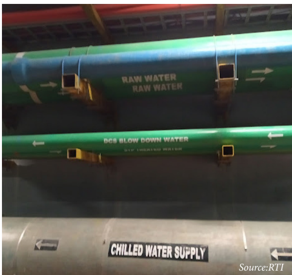
Figure 6.7: Underground Utility Tunnel in GIFT city
