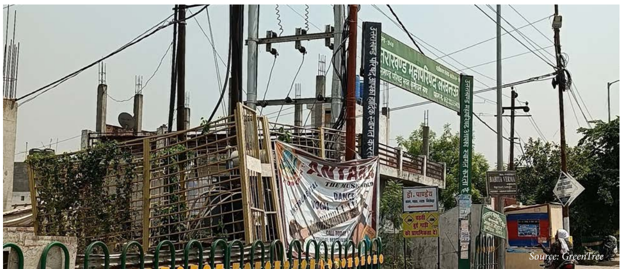
Figure 6.20: Status of Electrical Infrastructure in Lucknow
