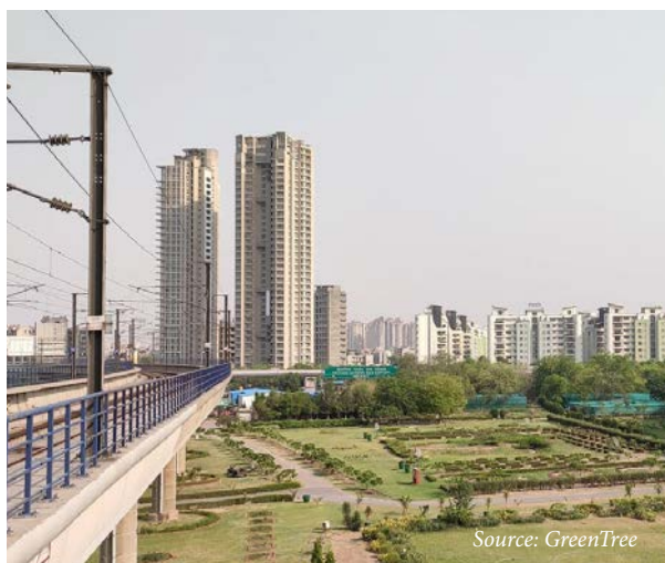
Figure 6.15: Urban infrastructure in Noida
