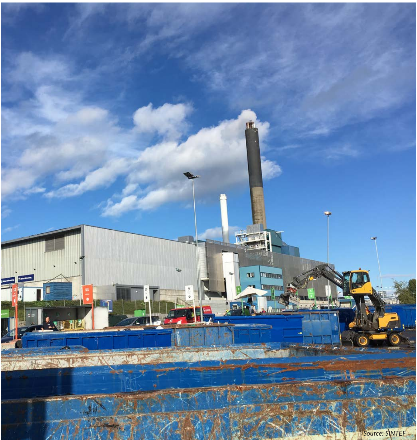
Figure 2.2: A modern WtE plant in Oslo
